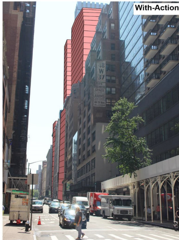
Facing east from W 37th Street east of 6th Avenue towards projected development sites 53 and 54.
