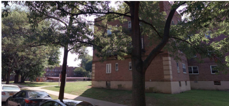
Source: NYC DCP, Cyclomedia Street View, Aug. 23, 2024
