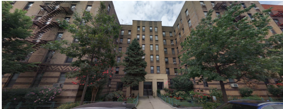
Source: NYC DCP, Cyclomedia Street View, Aug. 17, 2024
